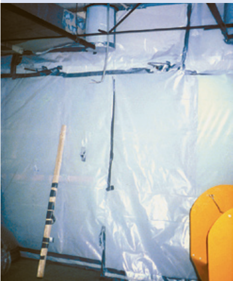
Photo 8: Full containment on large job
